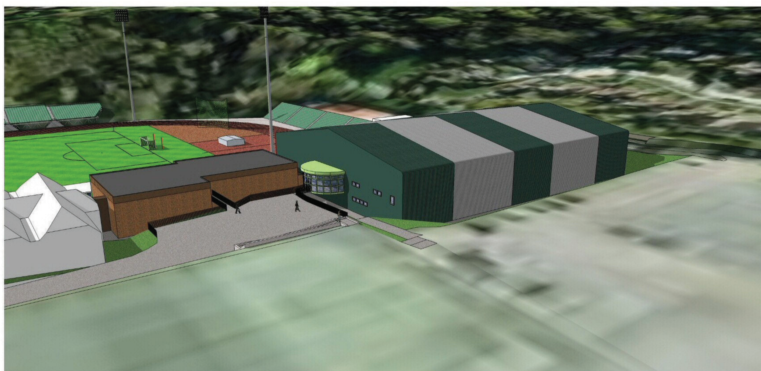
Existing Site View
